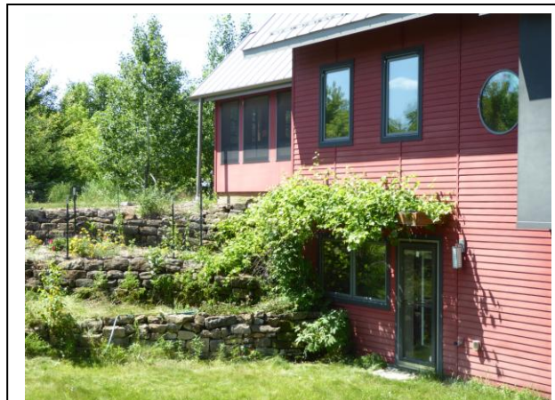
South side of home showing shade of overhang, and green awning holding grape vines for food and cooling; retaining walls, recovered from old farm home foundation, hide 1,000 gallon cistern with gravity feed faucet.
