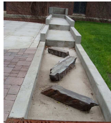
Trinity storm runoff system
